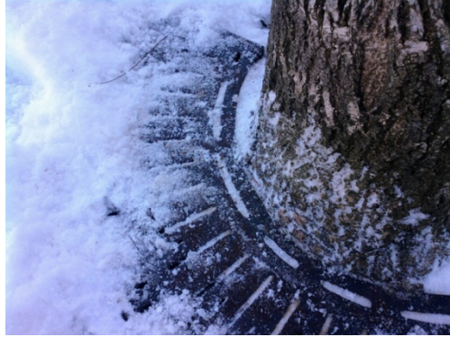
Figure 16: Tree trunk becoming swollen as a result of an undersized grate ring diameter. Taken by Kevin Boucher on 1/10/2011.
